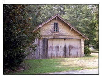
This garage was constructed about 1920 on the Shields-Ethridge farm in Jackson County (Piedmont Region). It has concrete block walls, wooden doors, and an unusual wood shingle design in the gable.
