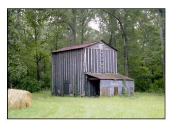
The photograph above shows a 1920s flue-cured tobacco barn in Effingham County with an attached shelter for the exterior furnace. The photograph below is a tobacco barn in Berrien County with wide overhanging sheds (shade skirts) for the stripping process. Both are located in the Central Coastal Plain.
