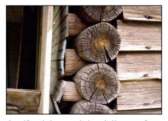
The saddle-notched corner on this log outbuilding is partially covered by weatherboard siding.
