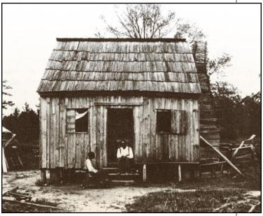
This 19th century dwelling was built with a mud-and-stick chimney, shown with its characteristic lean away from the wall of the house. Since the chimney was constructed of wood, it would be allowed to collapse away from the house in the event it caught fire. From McDaniel (1982:73).
