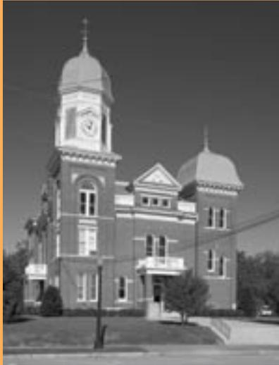
redwood to insure resistance to decay. Clock machinery was repaired and the original four clock faces were restored and a chime was incorporated. In addition, controls were added in the administrative offices that allow the time to be changed remotely.
