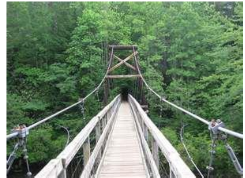
Swinging bridge over the Toccoa River, Benton MacKaye Trail
