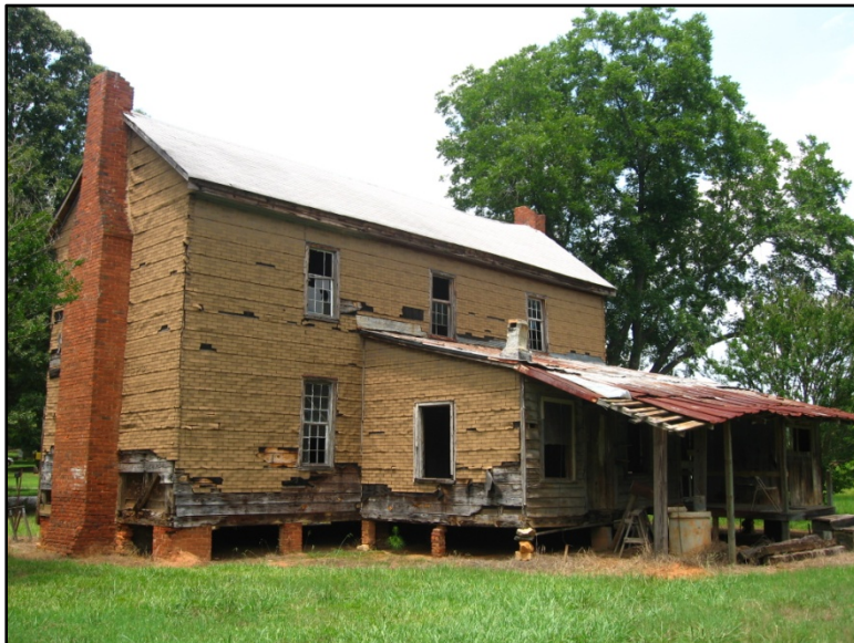
Figure 8 Rear elevation of the Cox House.
