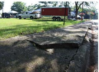
Picture 10: Cracked sidewalk in Forsyth
