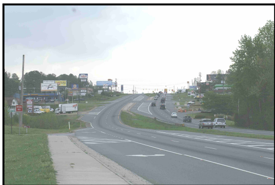
Figure 2-1: Cobb Parkway- North of Watts Drive
