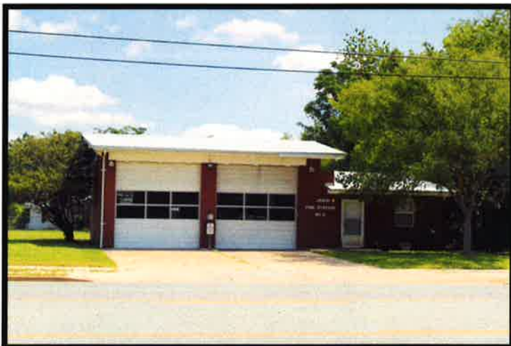
Newly renovated Jesup Fire Station #2
