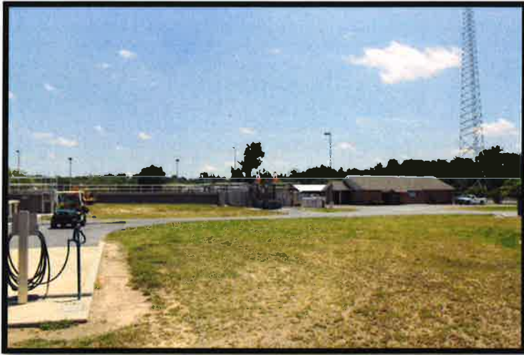
New Jesup Wastewater Treatment Plant
