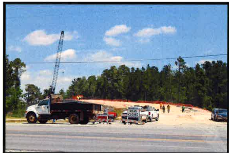
Georgia Highway 169 Overpass (Regional TIA Project) under construction
