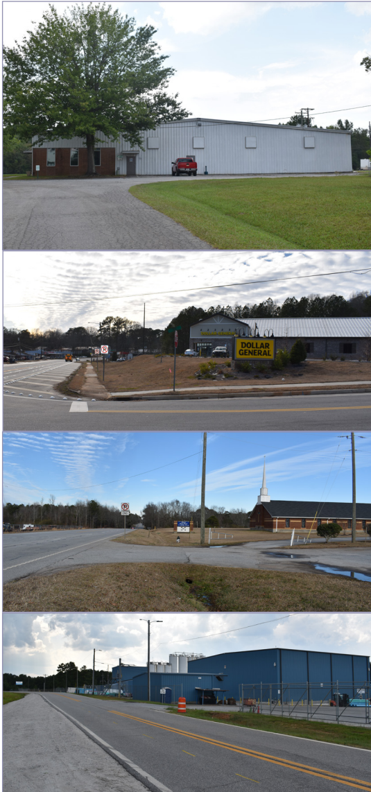
Figure 56. The Transport Quarter Character Area is mainly a mix of light industrial, commercial, office, and institutional uses. Note that additional heavy industrial uses (bottom image) may be allowable on a very limited basis, as described in the narrative.
