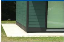
PH0T0 5 Concrete paver perimeter pest-resistant ground break. (Photo courtesy of the San Francisco Department of the Environment-*Pest Prevention by Design.*)
