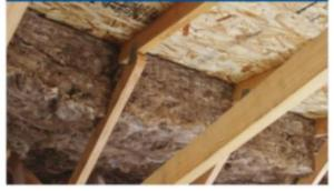
the underside of roof/attic sheathing. They obviously can't act as the water control layer, the air control layer or the vapor control layer. They can act as the thermal control layer if airflow through them is limited or controlled (*Photo 10* and *Photo 11*). We learned this with our "Thermal Metric Project."<sup>1</sup> In fact, the Thermal Metric Project showed that all cavity insulations functioned if they were combined with air control layers and if convection was controlled (*Figure 2*).
