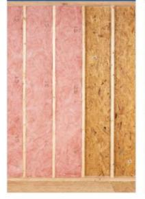
PROTO 11 Faced Insulation Batts. Airflow and convection can be effectively controlled by facers adhered to batt insulation. Note that faced insulation batts should have the facers installed to the face of the stud framing, not inset stapled. Inset stapling creates voids and air channels that can lead to convective loops and a loss of thermal resistance.
