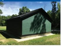
**PHOTO 4** Concrete skirt perimeter pest-resistant ground break.
