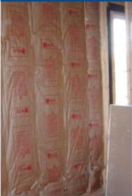
FIGURE 2 Cavity Insulation Airflow Pathways. There are 12 possible airflow pathways that can reduce the thermal resistance of cavity insulations. Cavity insulations can act as effective thermal control layers. The Thermal Metric Project<sup>1</sup> showed that all cavity insulations functioned if they were combined with air control layers and if convection was controlled. Let me be specific and obvious. If batts are installed and fitted "tightly" without
