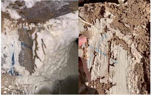
Picture 4. Images of the area in the SPF at Location 5 that provided visible evidence of termite activity on surface of SPF... left (outlined by the red box) and that same area exposed during foam removal.
