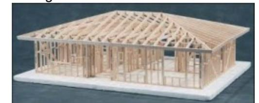
Figure 7-4: Example of a hip roof, which has more slopes than a traditional gable roof
