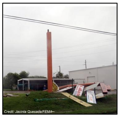
Figure 9-1: A freestanding sign that is damaged by a high wind can potentially cause damage to surrounding areas.
