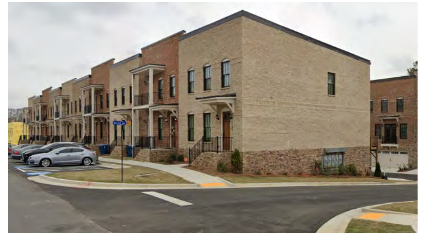
Brownstones at the Railyard – new attached housing
