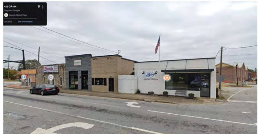
o Old buildings renovations as part of The Railyard in 2023
