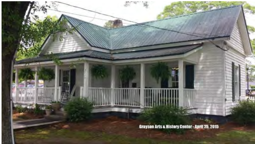
Kennerly-Cox House (a.k.a. Arts & History Center)
