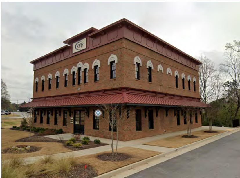
o VPR Real Estate Office Building at The Railyard
