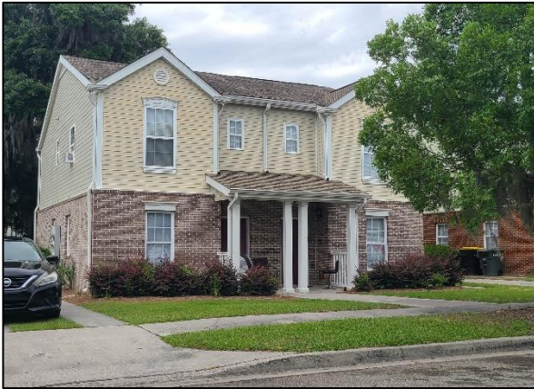
Existing duplex building
