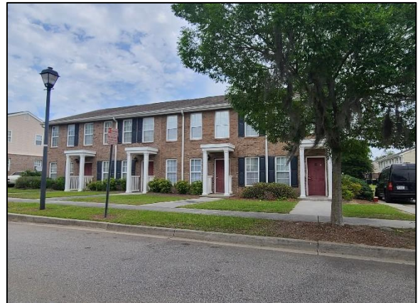
Existing townhome building
