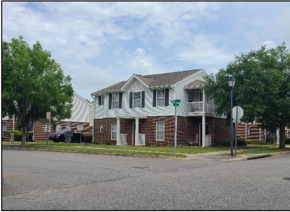
View of subject property site along Park Avenue
