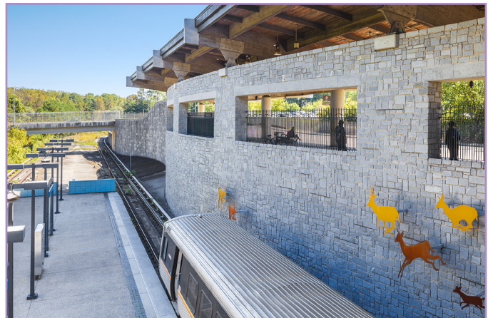
Figure 13: Indian Creek Station is the terminal station on MARTA's East-West heavy rail line, and an anchor for the Indian Creek Regional Activity Center
