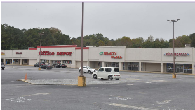
Figure 1: Many older strip-center developments, such as this plaza along Memorial Dr, are declining and in need of redevelopment
