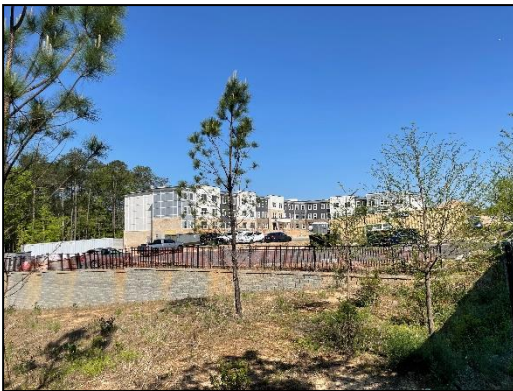
Phase II and south side of Phase III from Phase I
