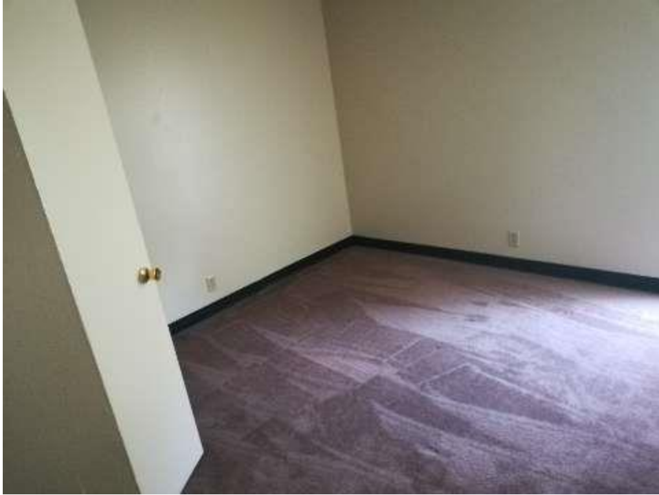
View of Typical Bedroom
