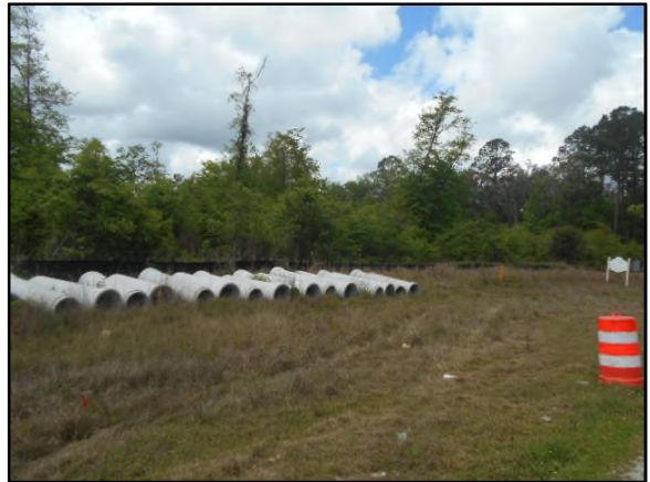
Site facing southwest from Laurel Island Parkway.
