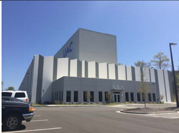
New manufacturing facility located east of the site
