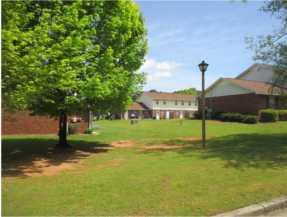
View to the North
