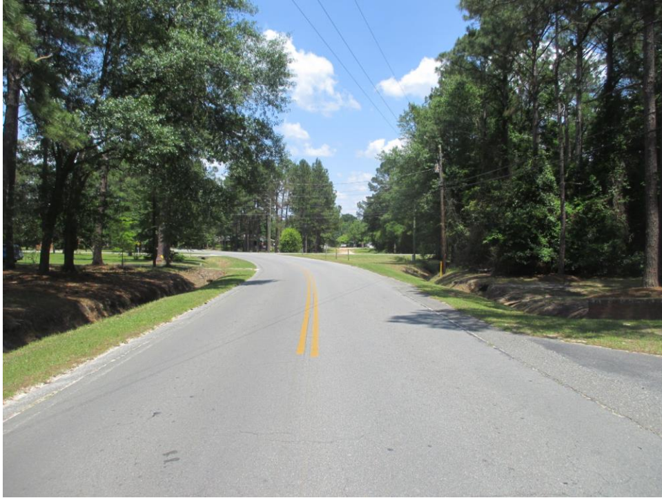
View to the North
