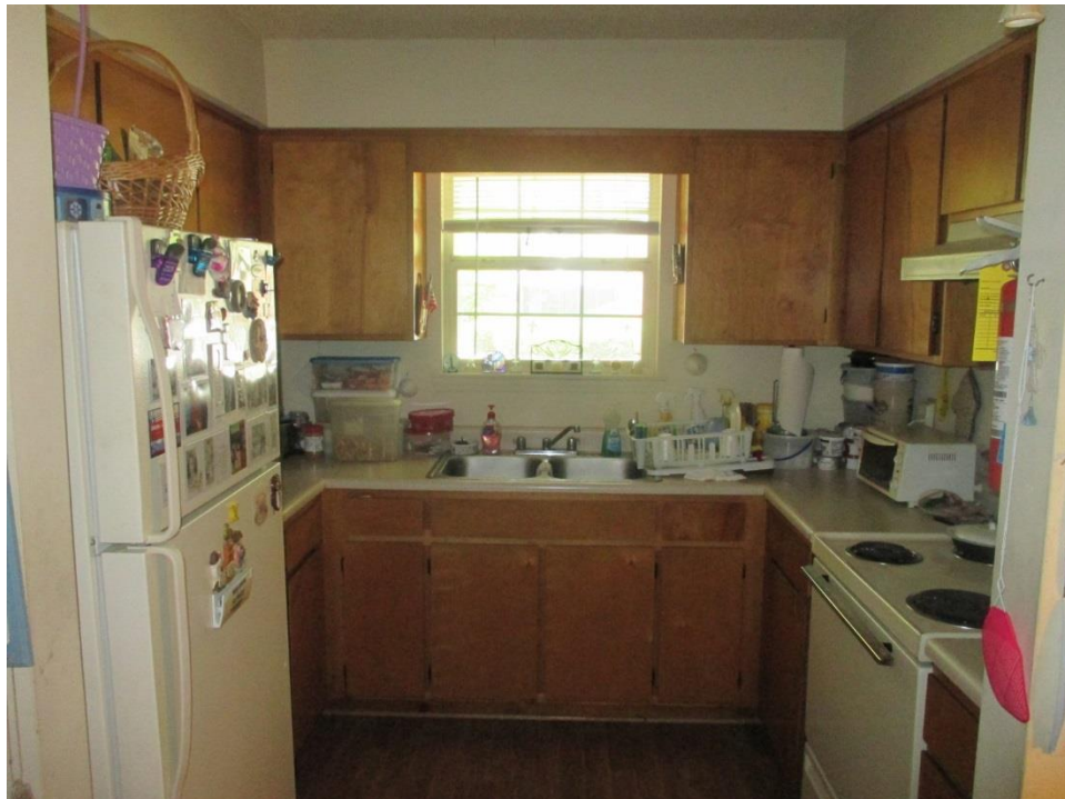
View of Kitchen – Two-Bedroom Unit
