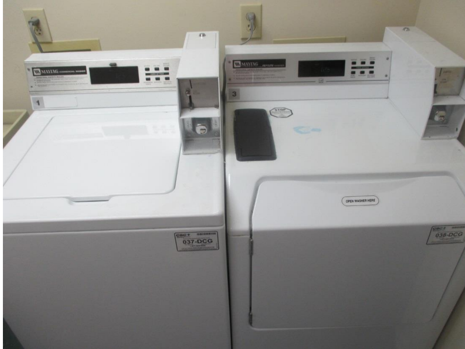
View of Laundry Facility
