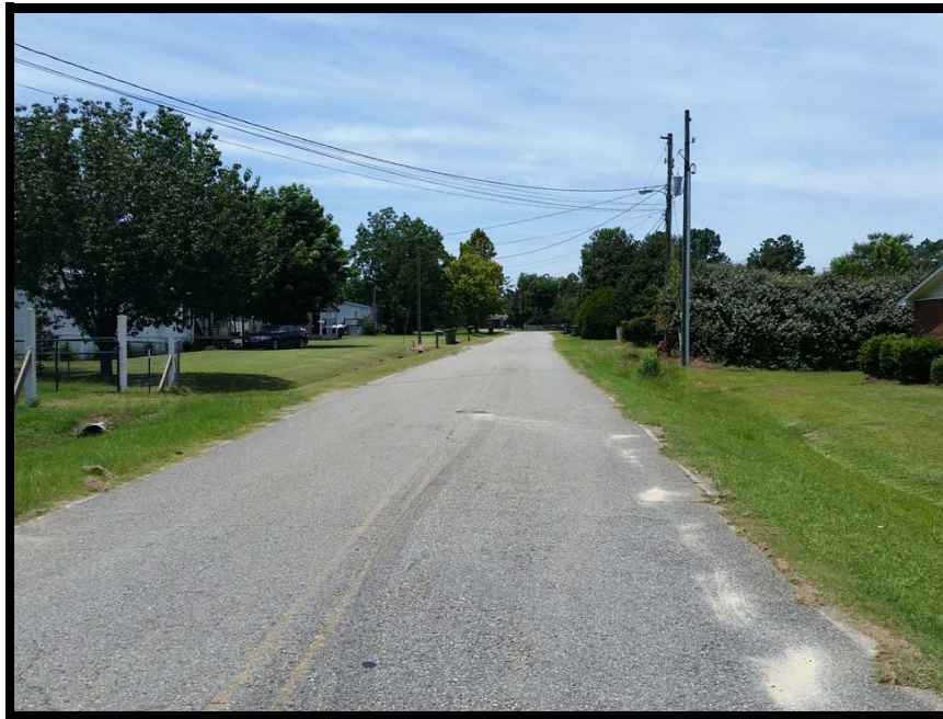
Streetscape- West View of Spinks Drive
