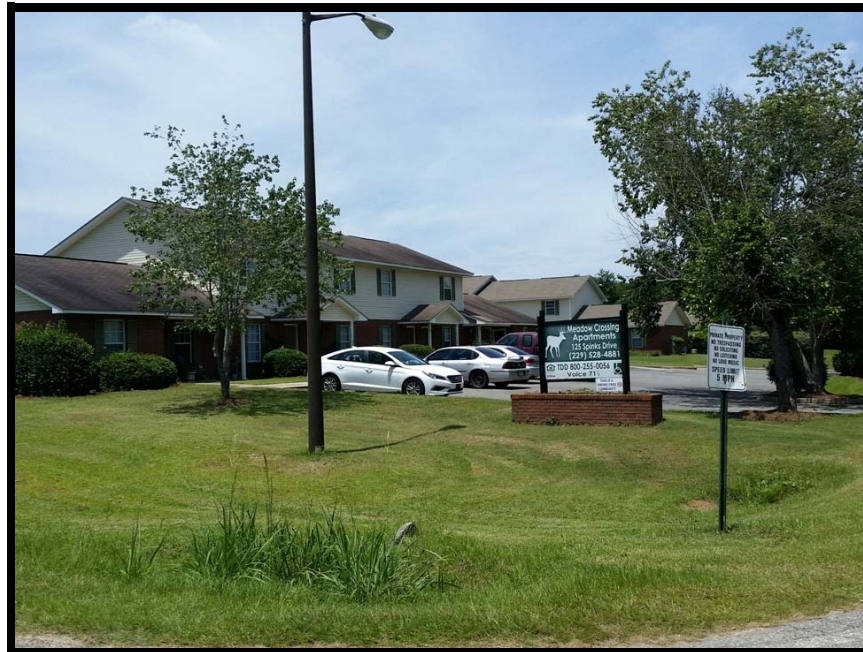
View of site from the southeast
