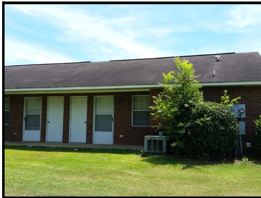
View of site from the north
