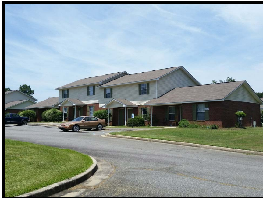
Typical Building Exterior
