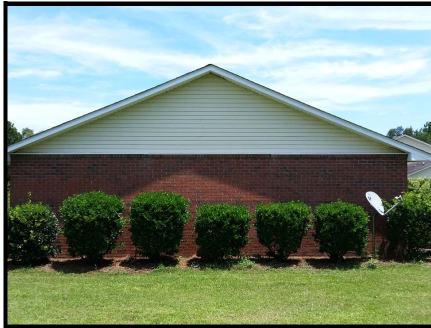
View of site from the west
