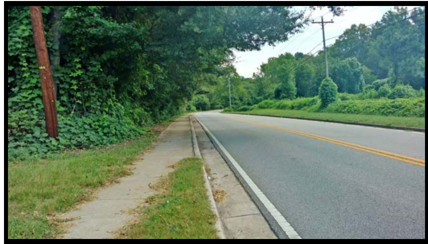
Streetscape: view facing east on Jefferson Street
