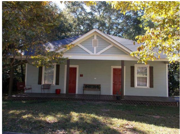
Typical single family housing in Subject's neighborhood.
