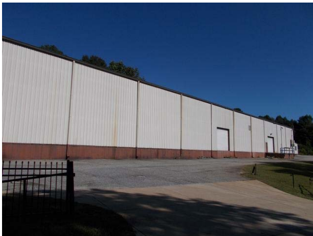
Warehouse located immediately to the west of the Subject (Jefferson Street Extension)
