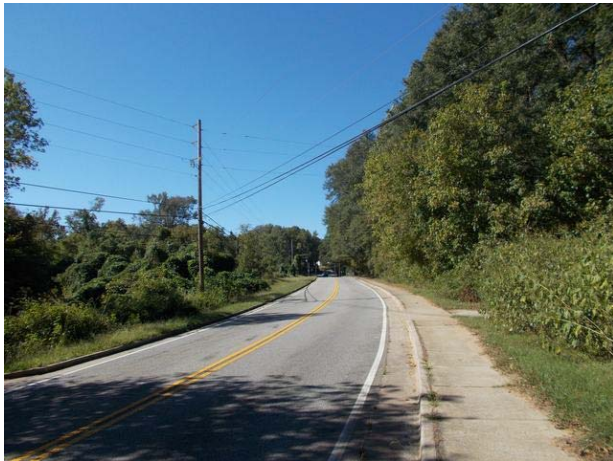
View from Subject site (Jefferson Street Extension) facing west
