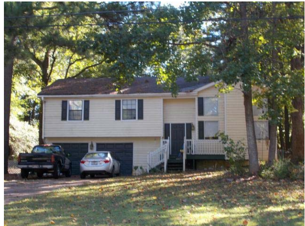
Typical single family housing in Subject's neighborhood
