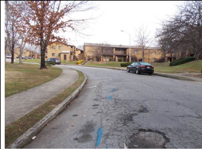
VIEW EAST FROM SUBJECT
