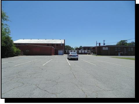
(1) Site entrance, Vineville Road, north to south.
