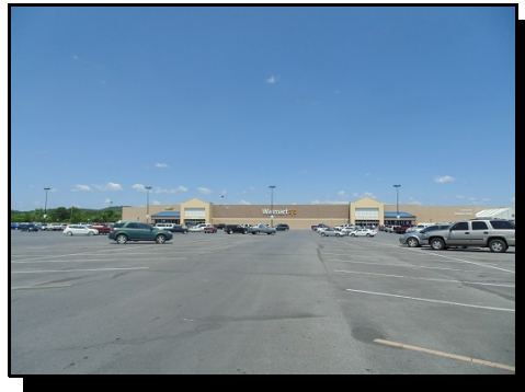
(12) Walmart Supercenter, 1 mile south of site.
