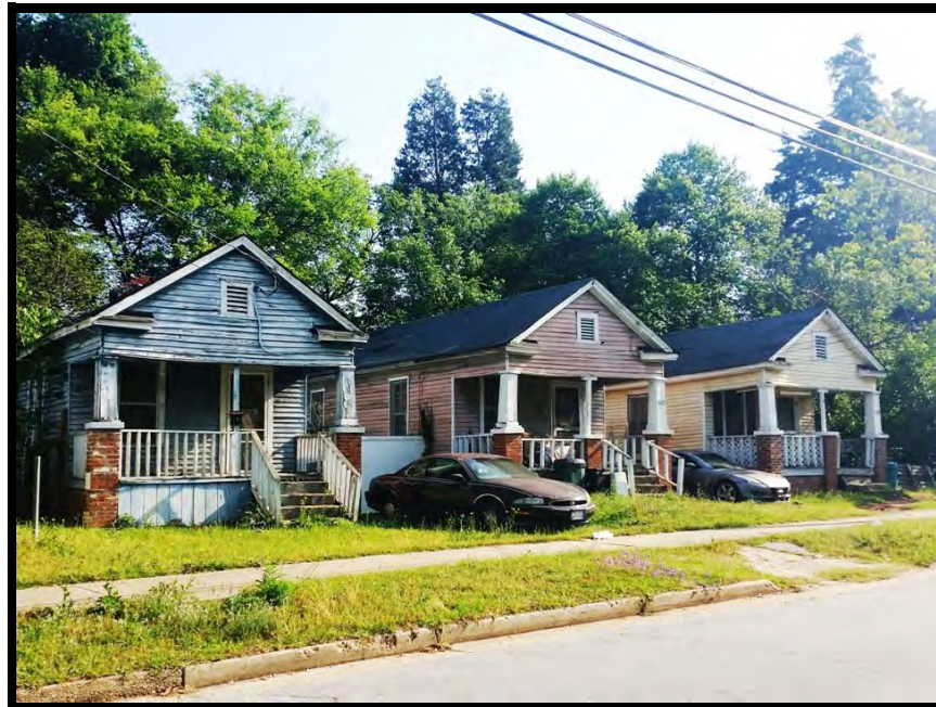
Typical homes in subpar condition southwest of site
