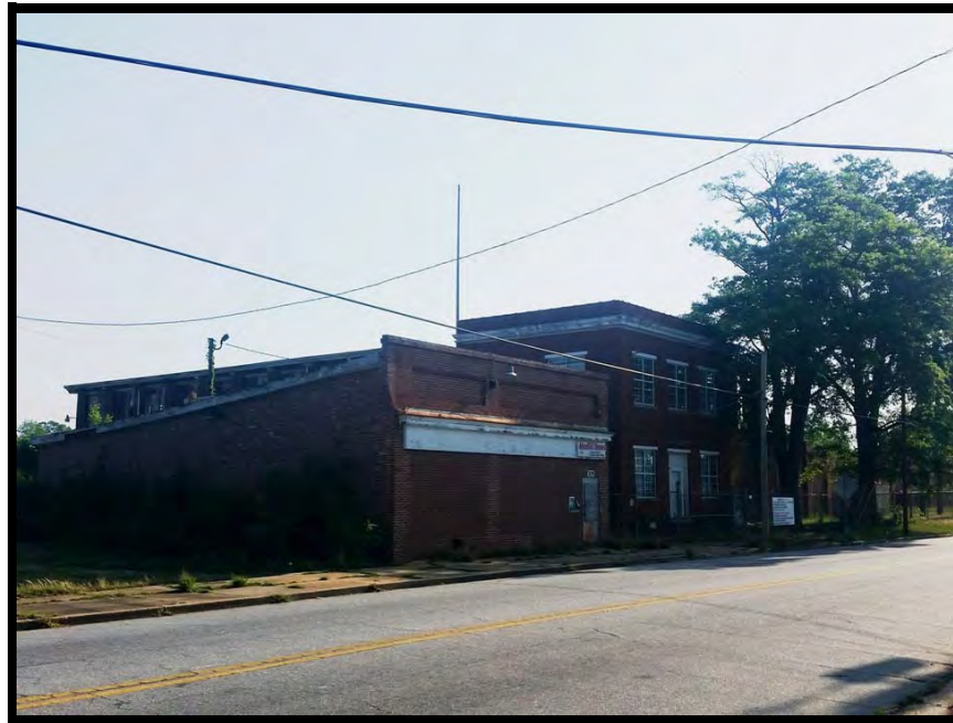
View of site from the southwest
