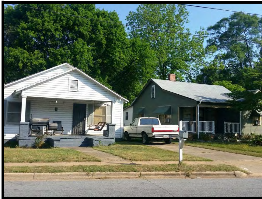
North view from site
