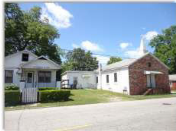
St. Sinai Baptist Church to the south.
