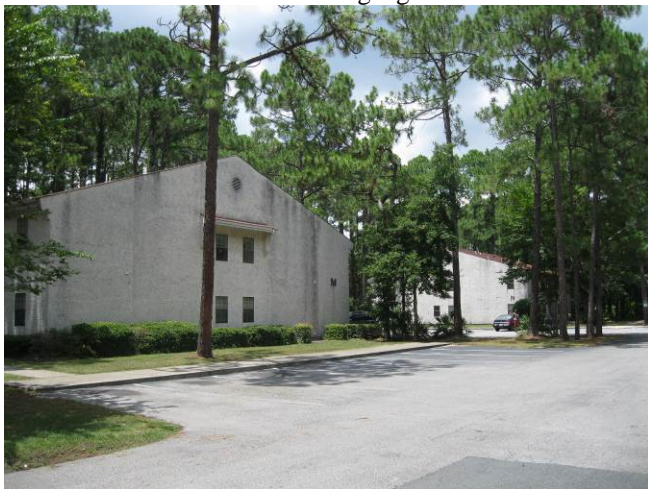
Exterior and parking
