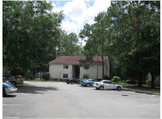
Exterior and parking
