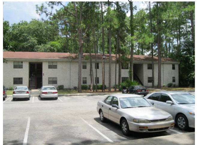
Exterior and parking
