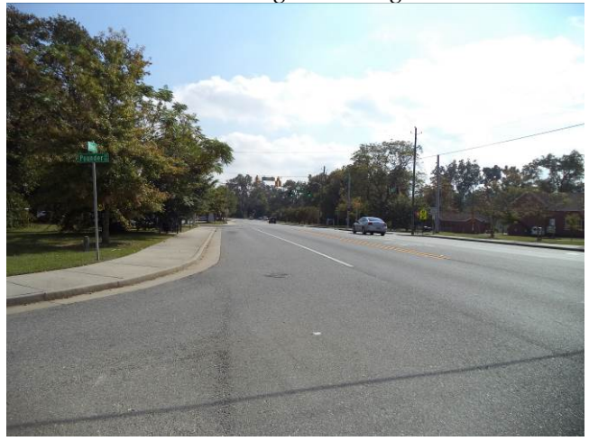
View south along Wheaton Street
