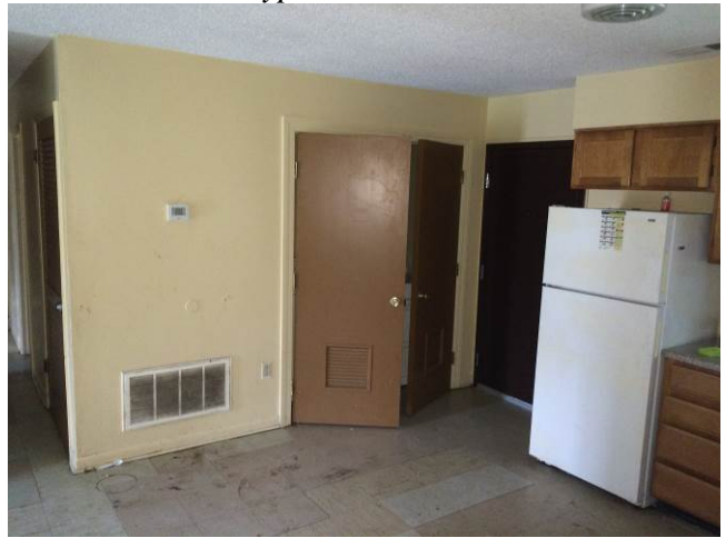
Typical washer/dryer closet
