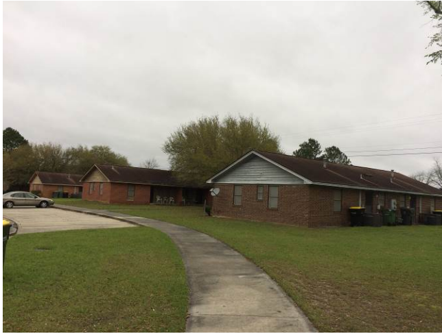
Site B exterior
