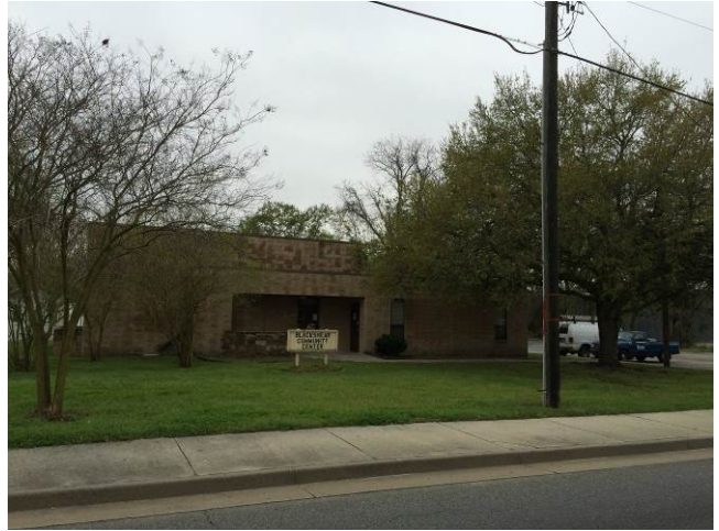
Blackshear Community Center along Wheaton Street
