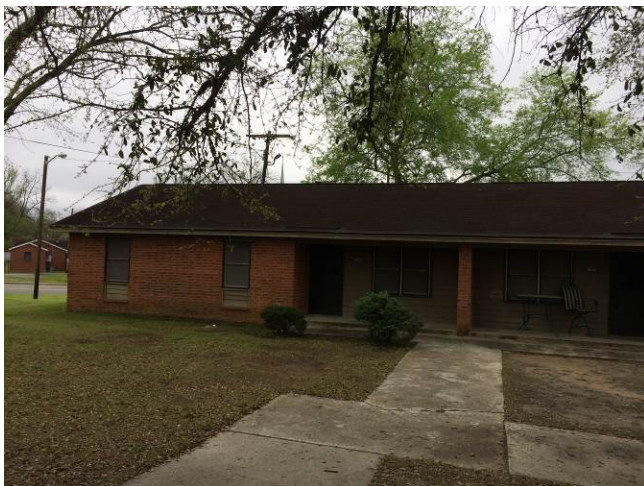
Site B exterior
