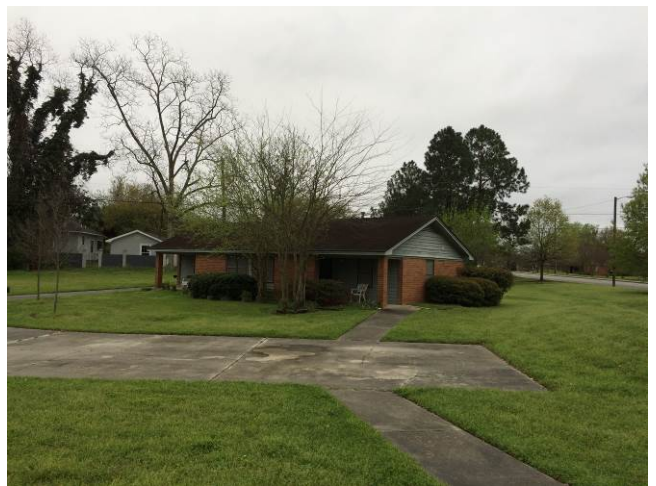
Site B exterior
