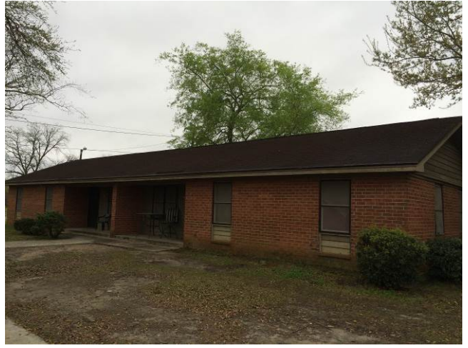
Site B exterior
