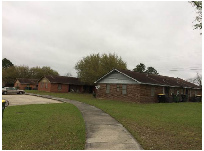
Site B exterior
