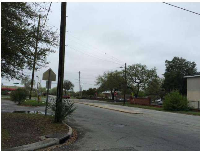
View south along Randolph Street
