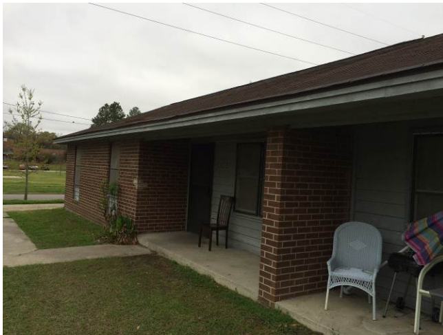
Site B exterior
