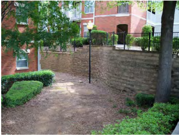
View Into Courtyard / Retaining Wall
