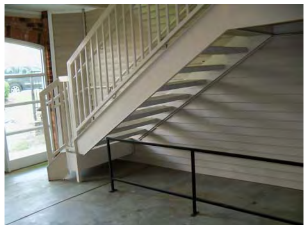
Stairwell To Apartments
