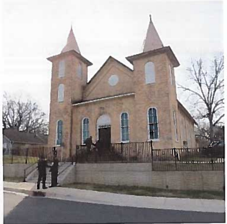
One of the architectural elements that is present at Bethel AME Church are its asymmetrical towers. One tower includes a cast iron bell that was rung as guests arrived.
