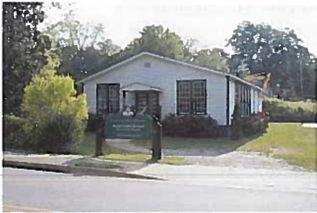
The Acworth Rosenwald School is located on Cherokee Street, just below Bethel AME Church. It is adaptively reused today as a community center and is a local destination for special events. The building is owned by the City of Acworth, a major partner and steward for the building. Photo by Jeanne Cyriaque
