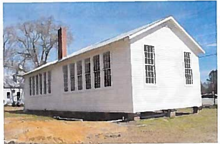
Each classroom in the Barney School features clusters of six banks of nine-over-nine windows. Photo by Jeanne Cyriaque
