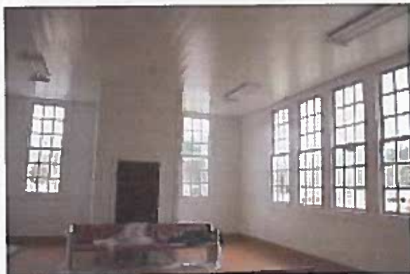
Today, a bathroom was installed in the rear classroom.
