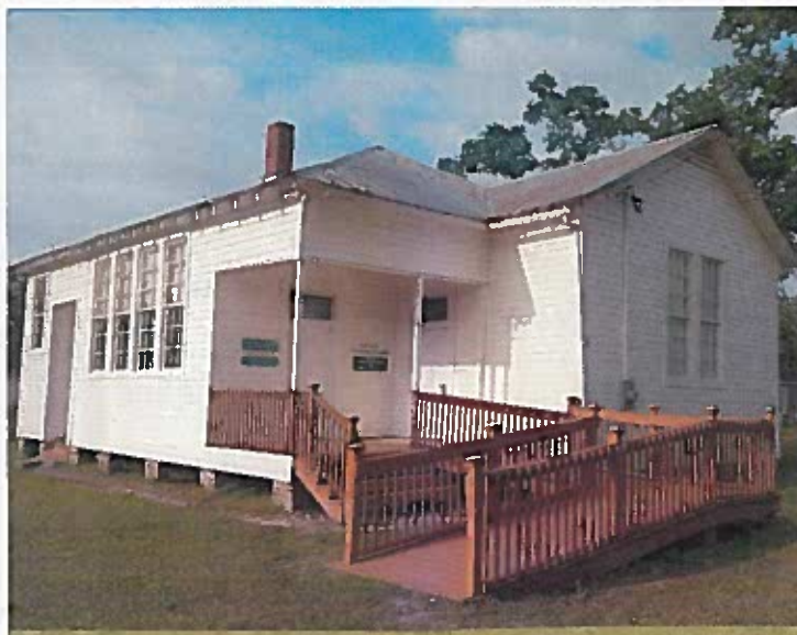
Barney Colored Elementary School was constructed in 1932 and served this rural community until 1959. It was preserved by the Morven Rosenwald Alumni Association.
