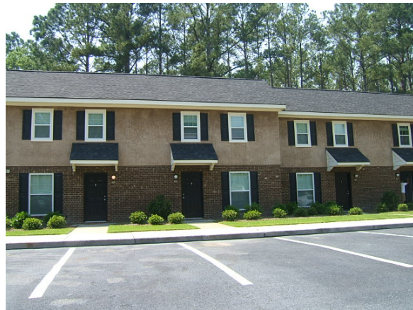
Mission Ridge Apartments bordering the subject site to the south
