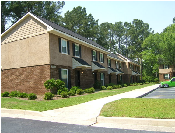
Mission Ridge Apartments bordering the site to the south
