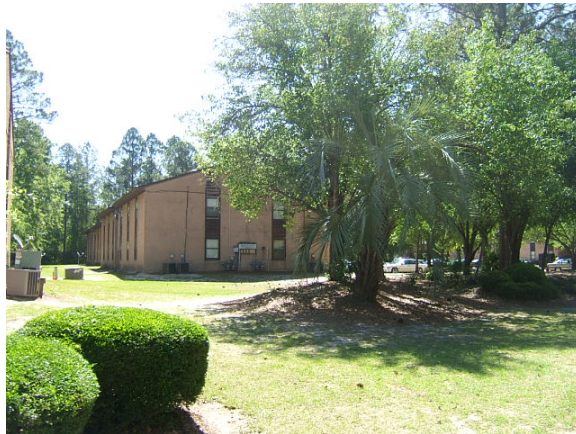
View of apartment buildings and circular parking lot on the southern end of the subject site
