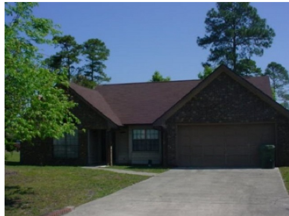
View of a single-family home northeast of the site
