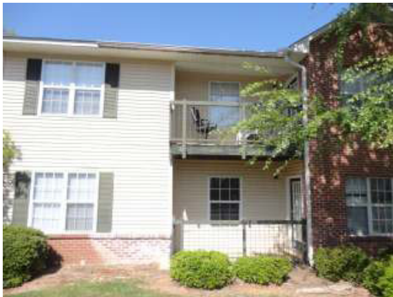
Exterior of subject property
