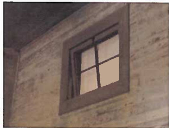
Breeze windows were located between the classrooms. Photo by Danielle Ross
