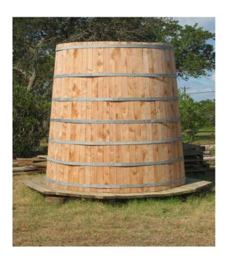
Figure 4.15 Wooden aboveground tank
