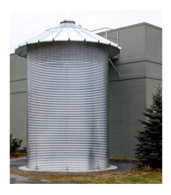
Figure 4-14 Corrugated steel tank
