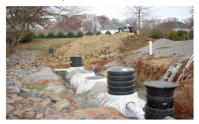
Figure 4.13 Below ground polypropylene tanks
