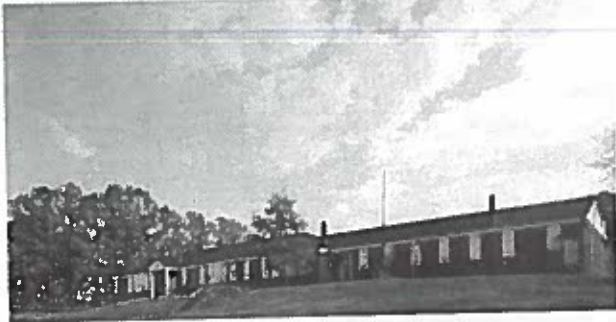
Classrooms and the auditorium were added to the north end of the building to relieve overcrowding. Photo by James R. Lockhart
