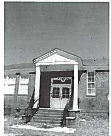
Entrances to Main High School have transoms above other windows and doors. Photo by Jeanne Cyriaque
