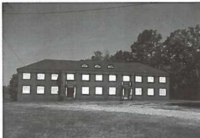
The Women's Dormitory is one of the historic buildings that remain from the State Teachers and Agricultural College era when the school was one of Georgia's three African American institutions in the University System of Georgia. The dormitory was constructed in 1936. Photo by Jeanne Cyriaque
