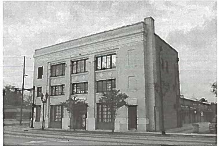
Penny Savings Bank is a community landmark building in the Laney-Walker Historic District. Its historic use was as a banking institution for African Americans and it is adaptively used for commercial purposes today.
