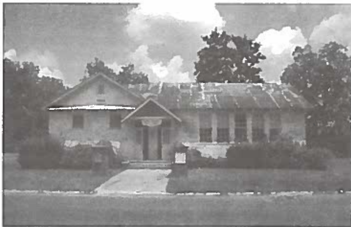
The Marian Anderson Library Rosenwald School in Blackshear, Pierce County, features brick columns at the entrance that were donated by alumni. The Blackshear Consolidated Men's Club operates youth mentoring programs at the Lee Street Resource Center, and is interested in preserving the library for community programs. The building was identified by the Okefenokee African American Heritage Society. Photo by Jeanne Cyriaque
