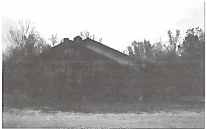
The Dock Kemp School was the only Rosenwald School built in Wrightsville, Johnson County. The building will require extensive preservation. It was identified by the Washington County Historical Society.
