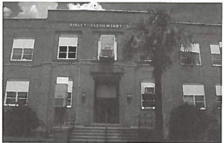
Risley High School (now Risley Elementary School) was built by the Public Works Administration under the New Deal in 1936. It is a redbrick, two-story building with stripped Classical details. Photo by Jeanne Cyriaque
