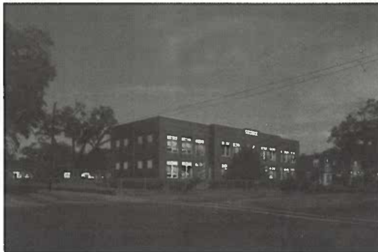
Colored Memorial School and Risley High School are two of the contributing resources on the Risley campus that were listed in the National Register of Historic Places on November 7, 2002.
