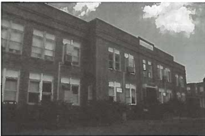
Colored Memorial School is a two-story, redbrick building. Constructed in 1923, the building has Neoclassical style details characterized by defining features including the original name panel "Memorial School 1922" over the front entrance.
