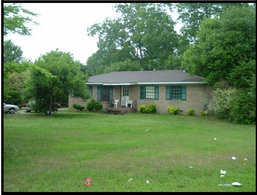
Single-family homes to the west
