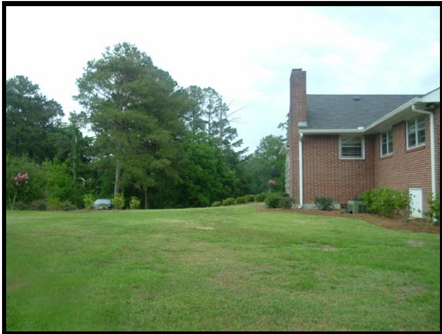
Westbound view of site
