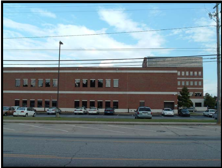
From Talbot Street facing east toward the Health and Human Services building
