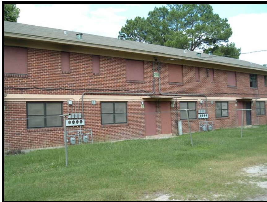
Back side of typical existing building
