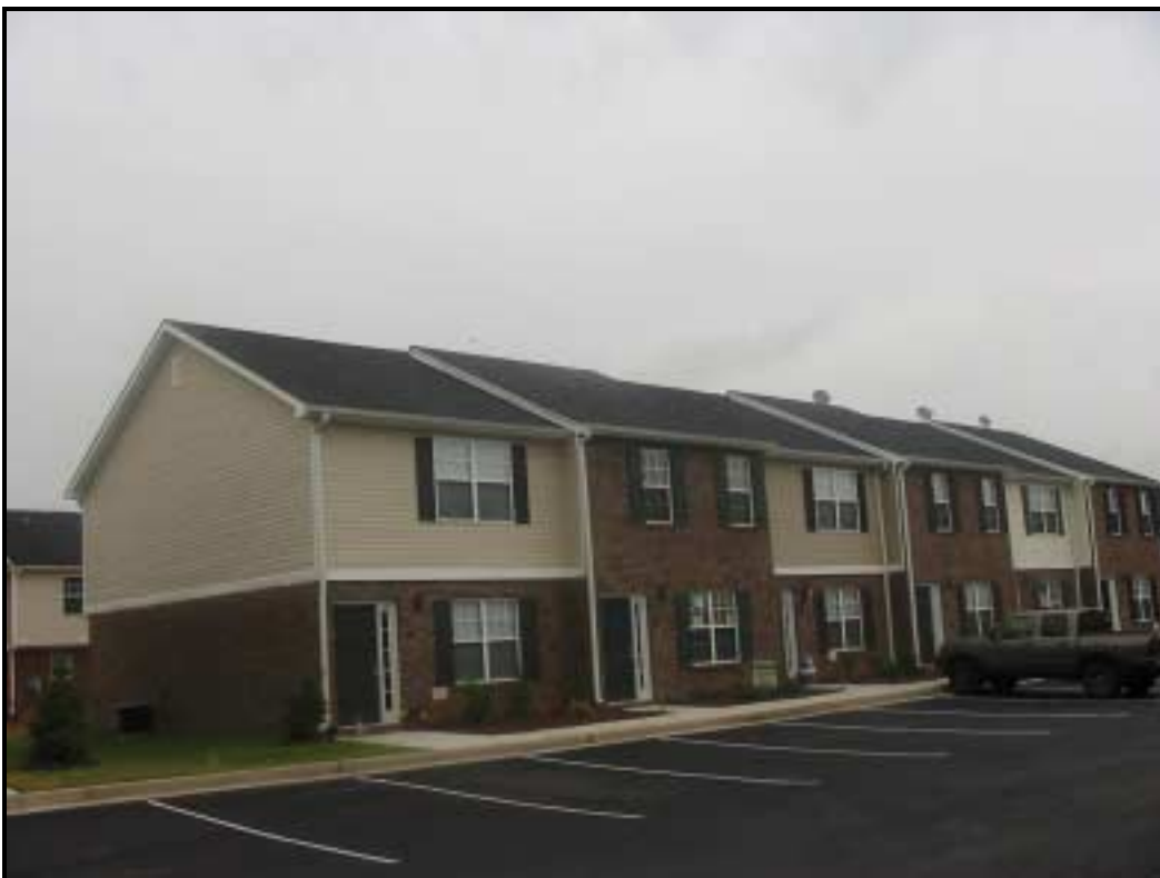
Princeton Glen Townhomes, under construction
