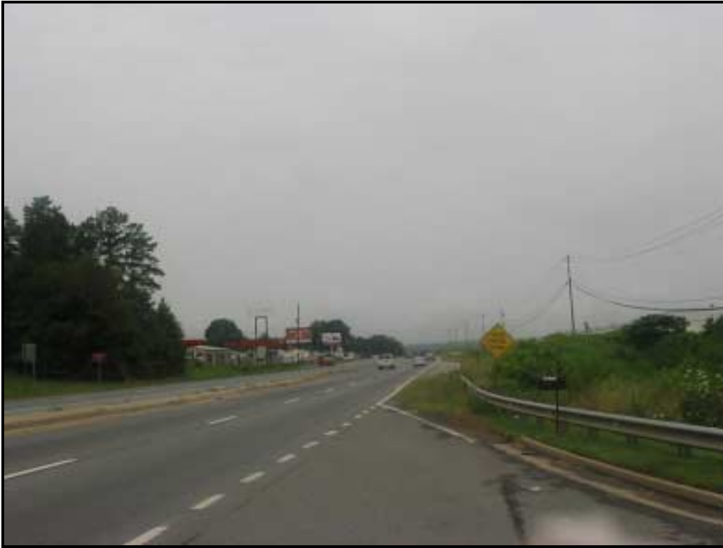
View of Highway 140 facing west from access road.
