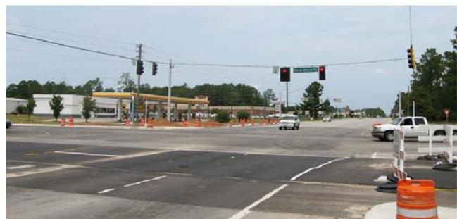
their intersections. Traffic lanes are very wide, with separate left turn lanes and median strips. Pedestrian and bicycle facilities are present but not connected to any nearby facilities, making accessibility difficult.
